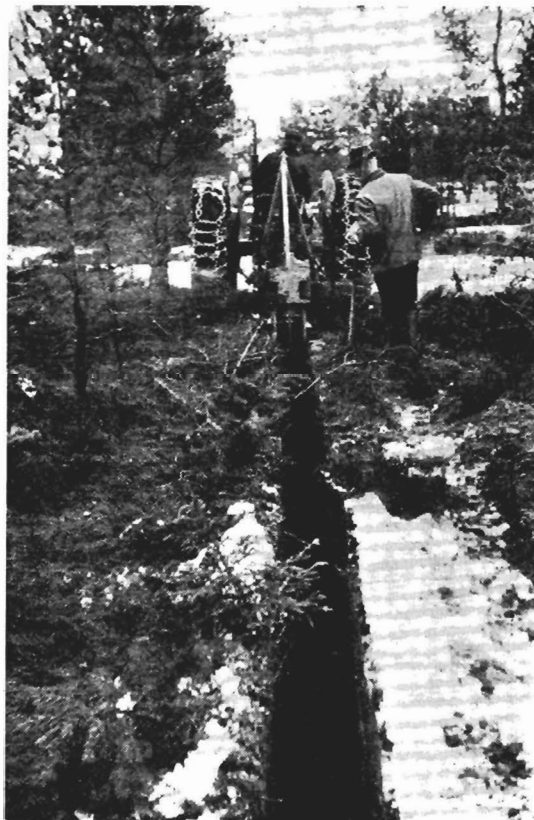
FIGURE 5. Preliminary draining in 1965 in a draining project of the Lapland agricultural engineering district in Muonio. In April, the snow had still to be removed from the top of the planned drain by a tractor. Photo M. Niskanen.
